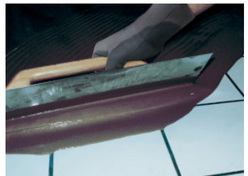
Application of Ultraplan with a metal trowel on an existing ceramic tile floor after the application of Eco Prim T Plus
