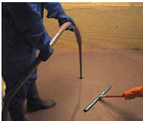
Application of Ultraplan with pump and squeegee
