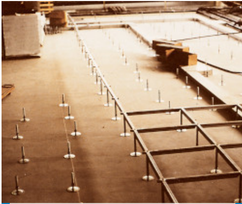
Slab levelled with Ultraplan ready for fixing a floating floor
