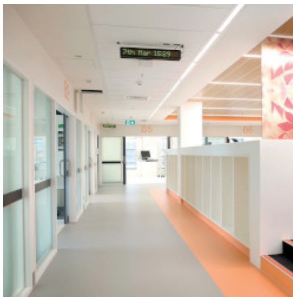
An example of an installation of linoleum on a surface levelled with Ultraplan - Victorian Comprehensive Cancer Centre - Melbourne - Australia
