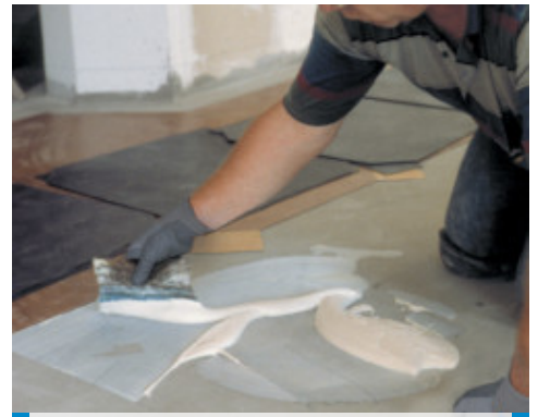
An example of an installation of inlaid PVC on a surface levelled with Ultraplan - CD 2 - Milan - Italy
